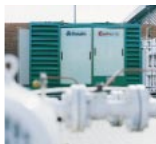
A typical fast fill compressed Natural Gas refuelling station supplied by CompAir.
