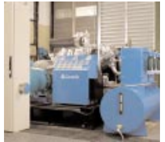
A pair of H5450 compressors fitted with membrane dehydrators supply air at 207 bar and -70 °C pressure dewpoint to 400 kV air blast circuit breakers. Didcot Power Station, UK's National Grid.
