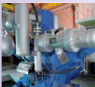
PET H5281 supplying oil-free high pressure air at Pysu Personal Care's PET bottle manufacturing centre.
