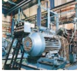
A bank of three CompAir H5450 compressors are dedicated to the compression of nitrogen used by Zotefoams in the production of packaging for the toy, motor, leisure and medical industries.
