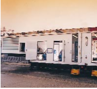
A mobile unit fitted by CompAir with H5436 compressors to supply blast air to the high voltage switch-gear of the National Grid during maintenance periods.
