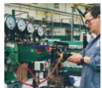
A CompAir 4 stage water cooled compressor and desiccant dryer provides quality clean air, essential for the calibration and testing of regulators manufactured by Gas Control Equipment Limited.
